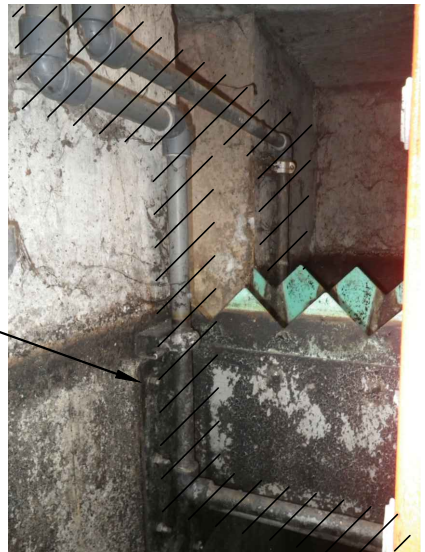
SLOTTED ADJUSTMENT BOLTS ON (E) LAUNDERS (TYP)
