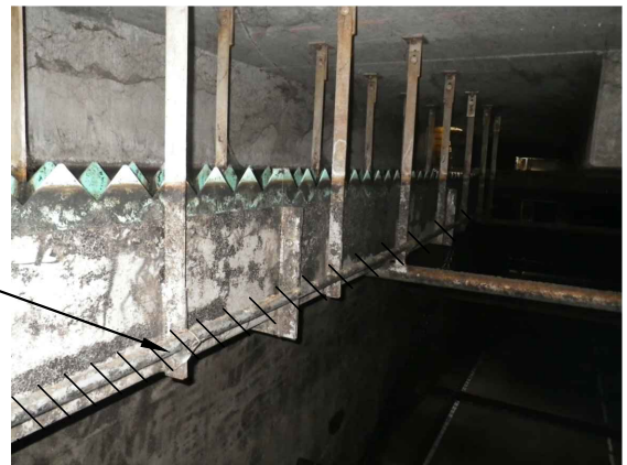
CONTRACTOR SHALL REMOVE (E) SPRINKLER PIPING AND PIPING SUPPORTS MOUNTED TO LAUNDERS.
