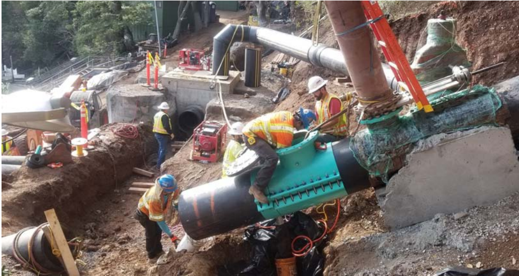
At work on a portion of the Treatment Plant Upgrade Project.
