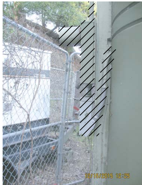
B PHOTO 2 - DEMOLITION ② NOT TO SCALE
