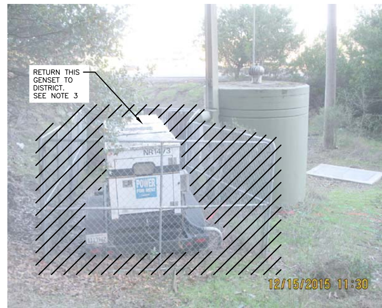
C PHOTO 3 - DEMOLITION ③ NOT TO SCALE
