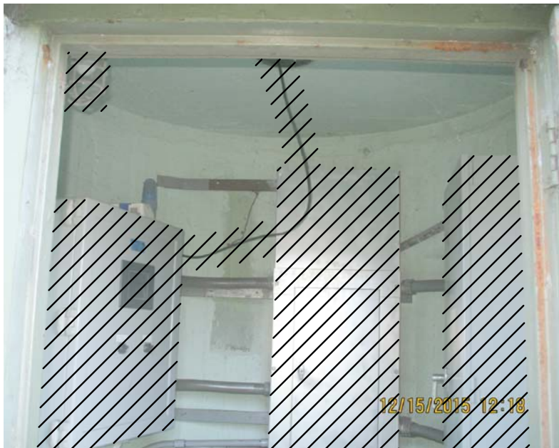
A PHOTO 1 - DEMOLITION ① NOT TO SCALE
