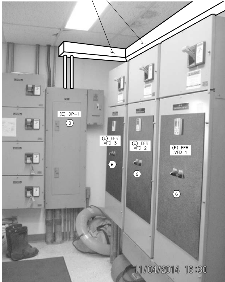
(E) DP-1 AND FFR VFDS B SCALE: NTS
