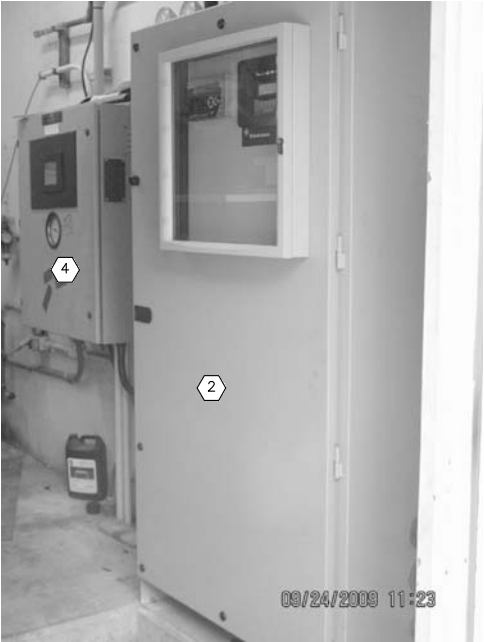
EXISTING ATS AND PLC-GEN B SCALE: NTS
