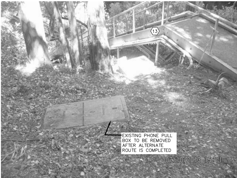
PHONE PULL BOX B SCALE: NTS
