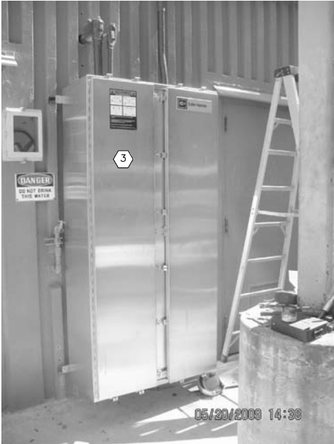
EXISTING POWER PANEL H-2 C SCALE: NTS
