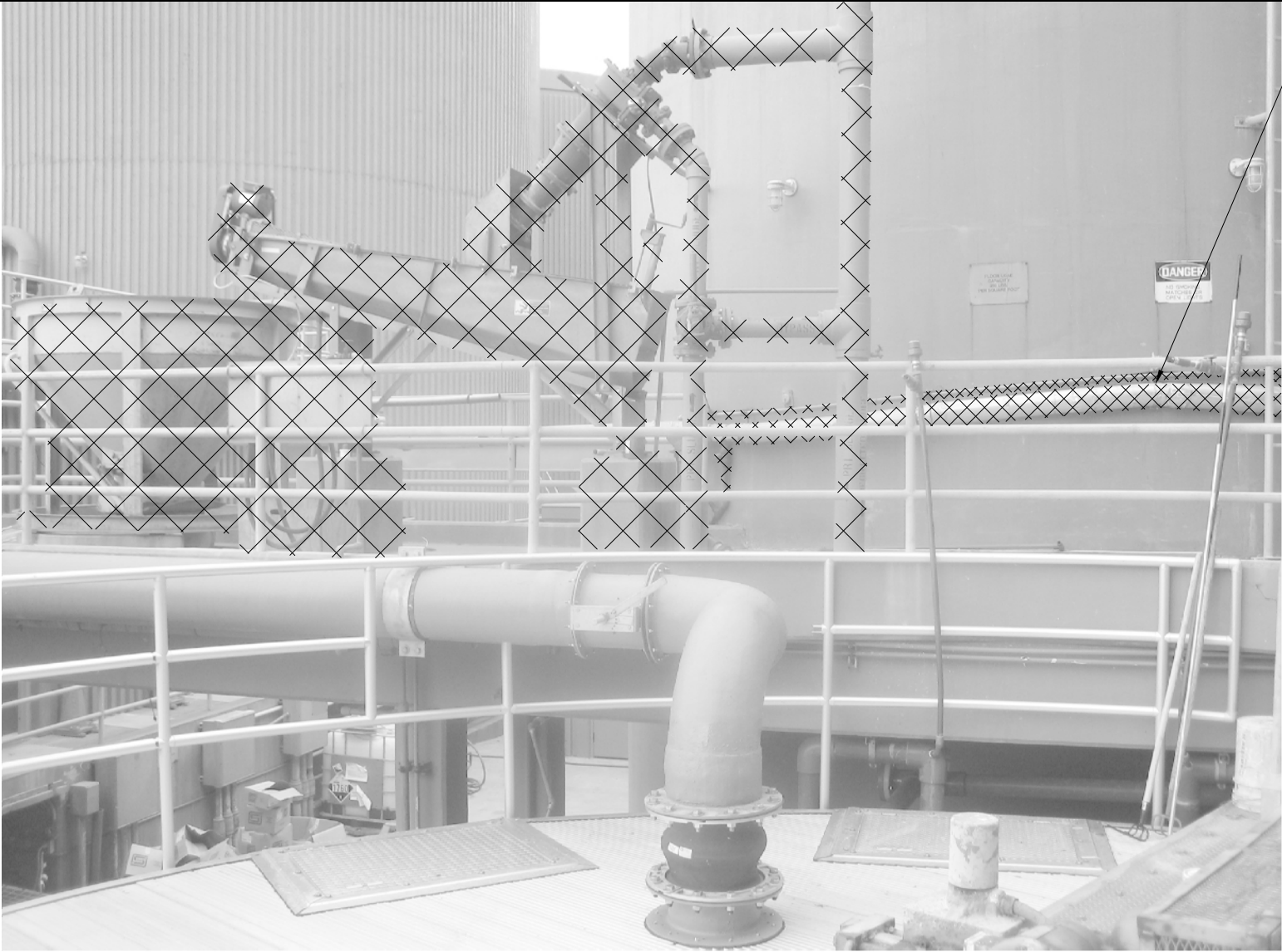
PHOTO (GRIT CLASSIFIER, HOPPER, PIPING AND APPURTENANCES) NOT TO SCALE P-3 M-1
