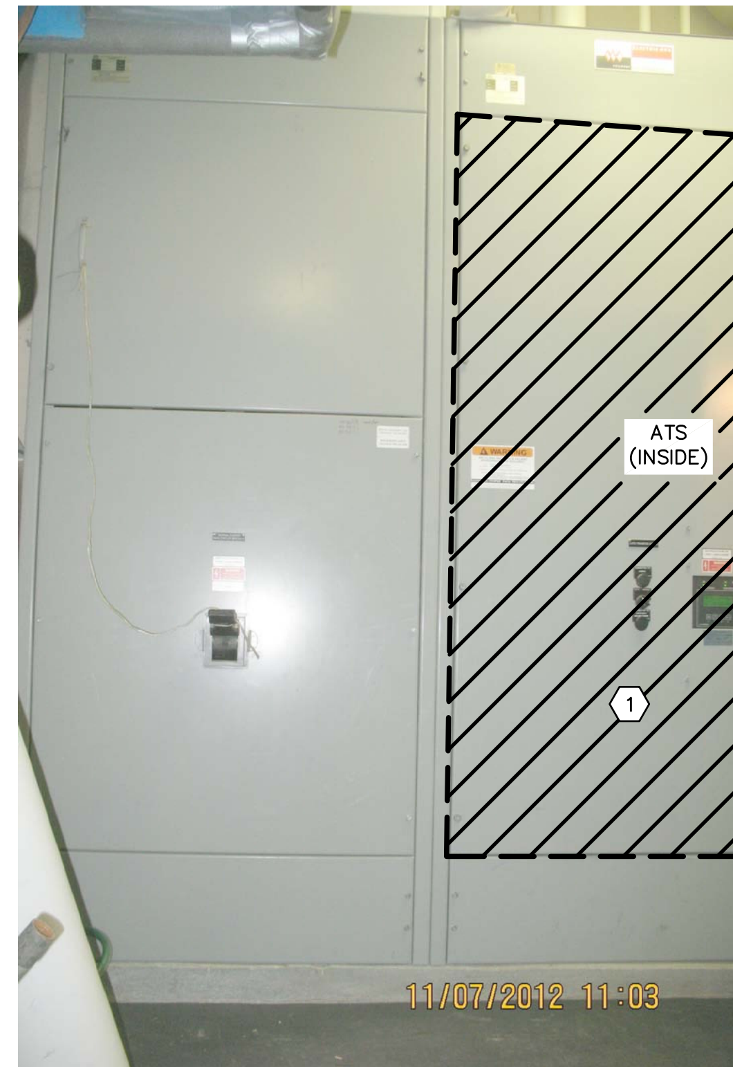
(G) DEMOLITION DETAIL 7 SCALE: NTS (E) MAIN ST ATS
