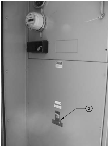
F NEW MAIN SERVICE BREAKER SCALE: NTS
