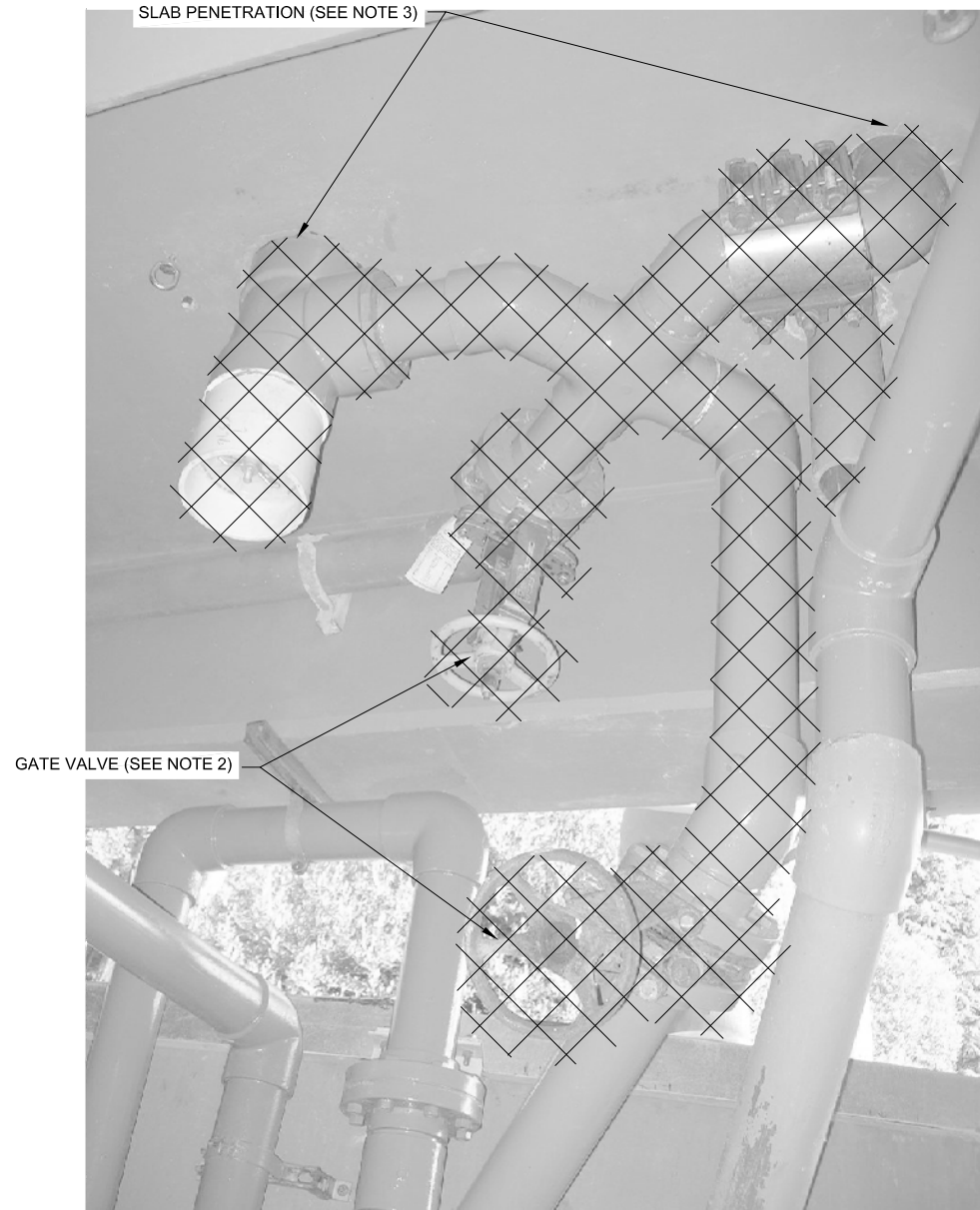
PHOTO P-3b (GRIT CLASSIFIER PIPING) NOT TO SCALE
