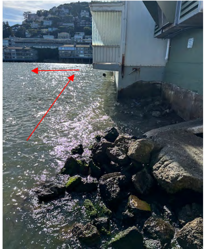
Photo 2: Inspection (pump station mainline route shown in red arrows)
