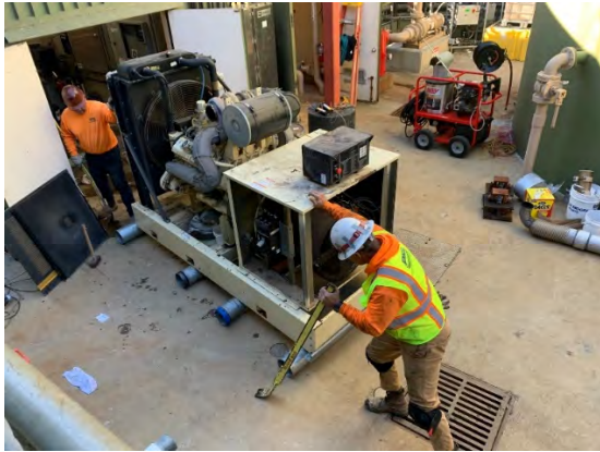
Old plant generator being removed.
