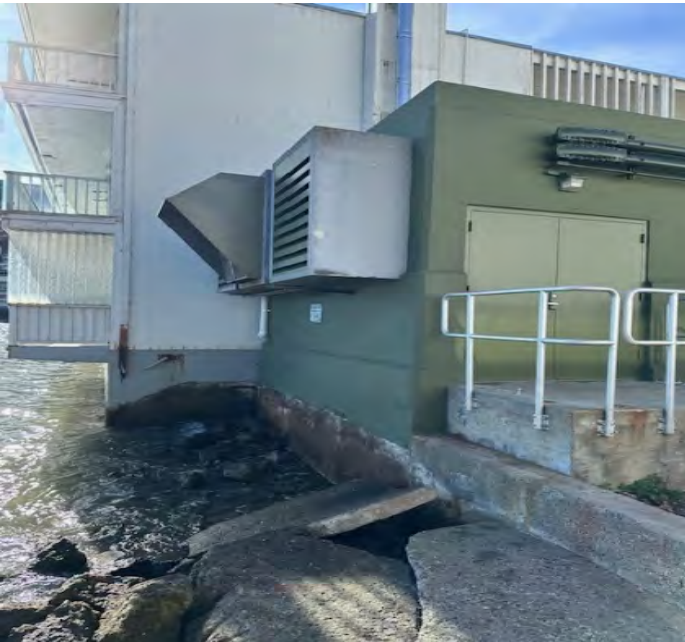
Photo 3: Inspection (pump station building)
