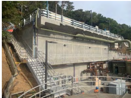
EQ Basin & New Stairs
