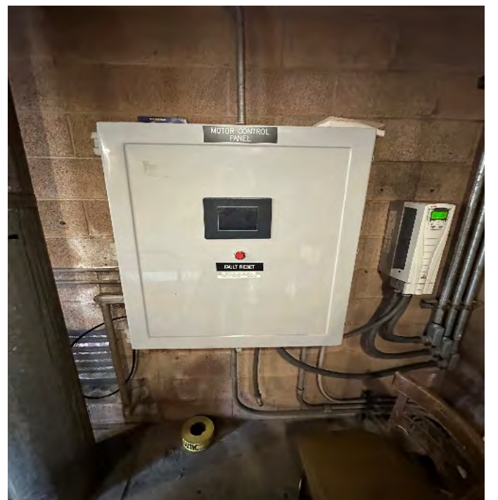
Photo 8: Inspection (operator controls)
