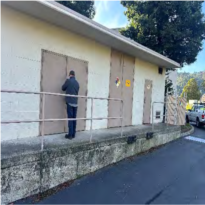
Photo 1: Inspection (pump station entry)
