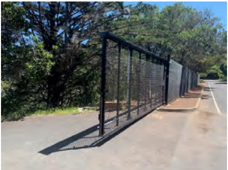
Treatment Plant entrance gate
