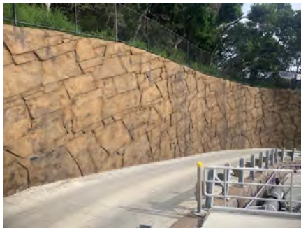
Completed Walls and Paving
