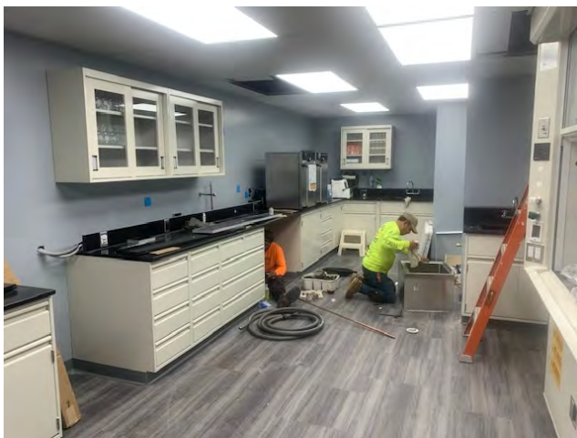
Final work being completed in new lab.
