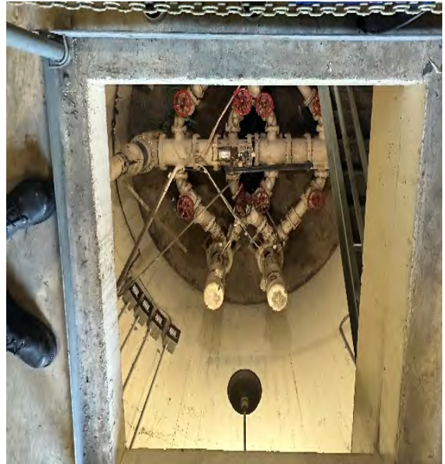
Photo 2: Inspection (pump station pump dry well)
