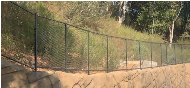
Fence installed around entire plant easement.
