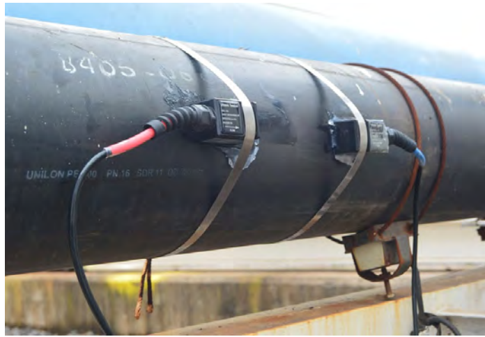
Example of a clamp on ultrasonic flow meter.
