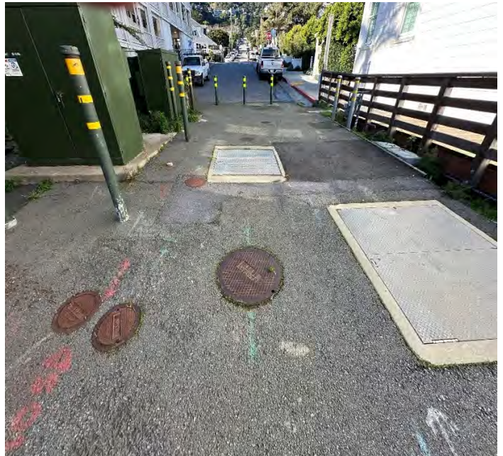
Photo 4: Inspection (pump station magnetic flow meter and bypass port)
