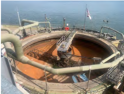
Clarifier prior to construction.
