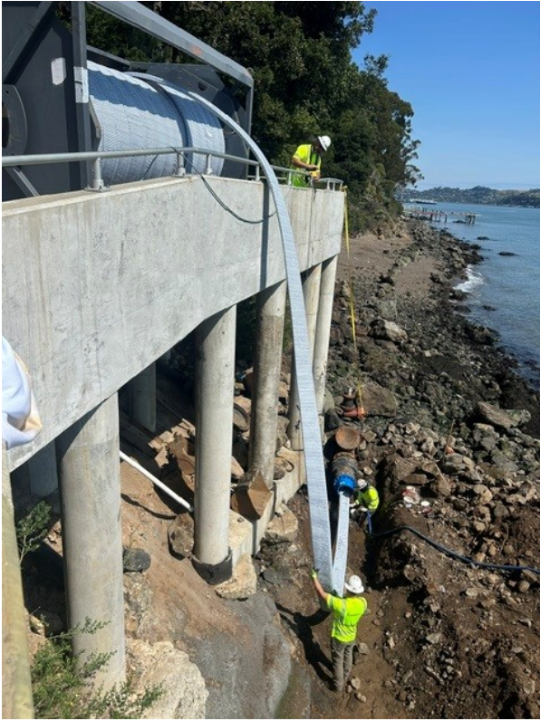
Liner being installed from Plant causeway.
