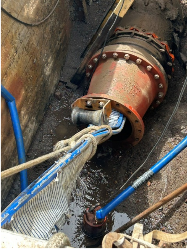
Liner being received at the Main St. PS
