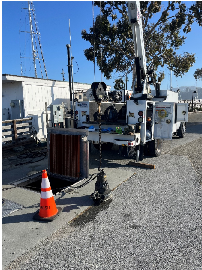
Pump #1 Removed from Wet Well
