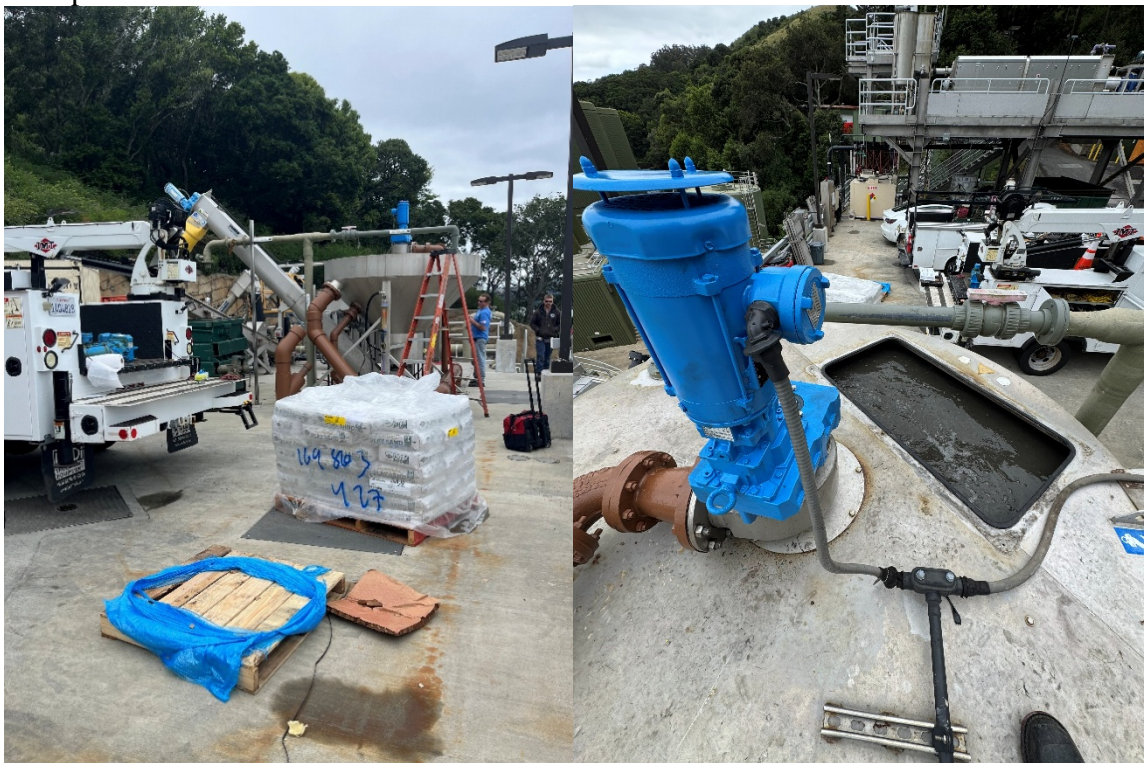
Crane Truck Used For Lifting
